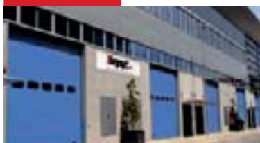
FACTORY AND TECHNICAL SERVICE
